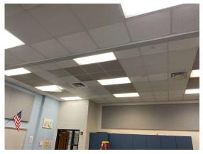
Examples of Wet Ceiling Tiles below AHU7/AHU8
